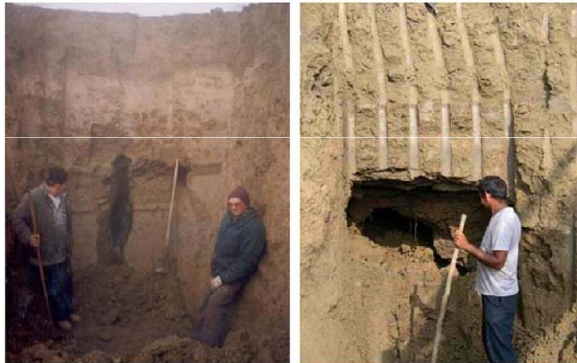
Fig. 1. Large voids found during a levee reconstruction that followed a breaching produced by piping due to the presence of animal burrows, Samoggia River, San Giovanni in Persiceto, Bologna, Italy (Mazzini and Simoni, 2008).
