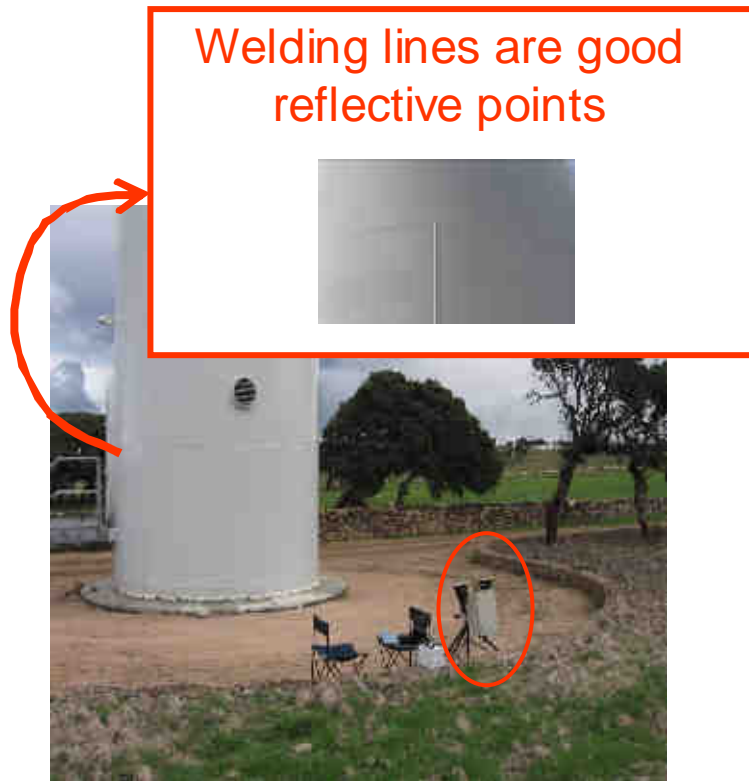
IBIS-S installed at the turbine pillar base (height 60m)
