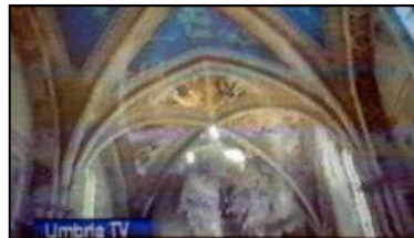
Sequence of the collapse of the vault of the Assisi Basilica during the 1997 earthquake
