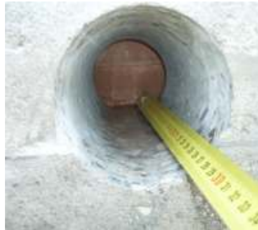
Coring and tests
