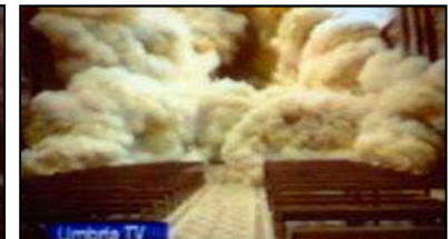
Sequence of the collapse of the vault of the Assisi Basilica during the 1997 earthquake
