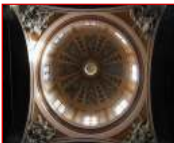
The dome (view from the bottom)
