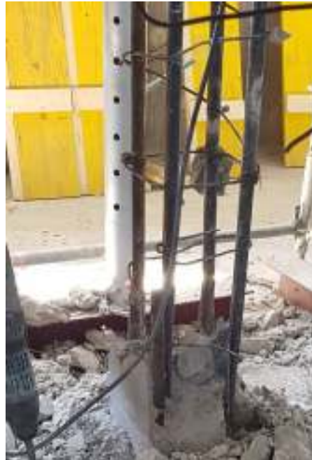
Typical steel reinforcement in columns
